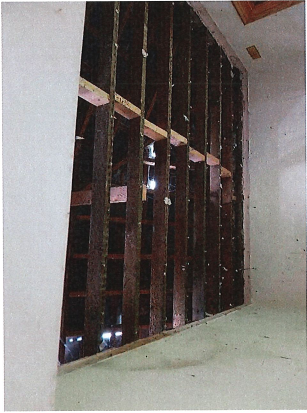
Fig. 6 – GF/02 - View ceiling joists
