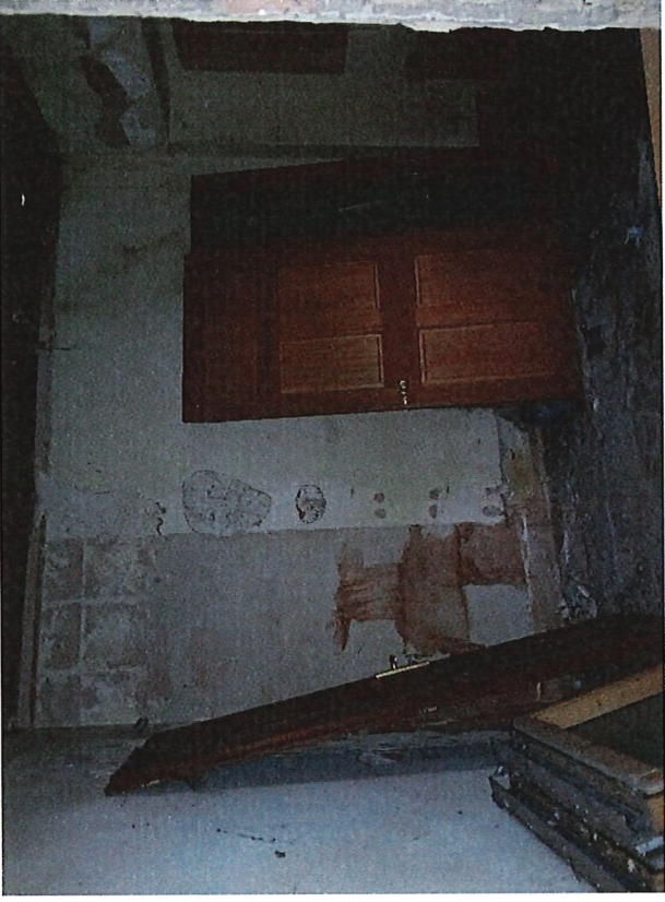
Fig. 7 – GF/04 - View south
