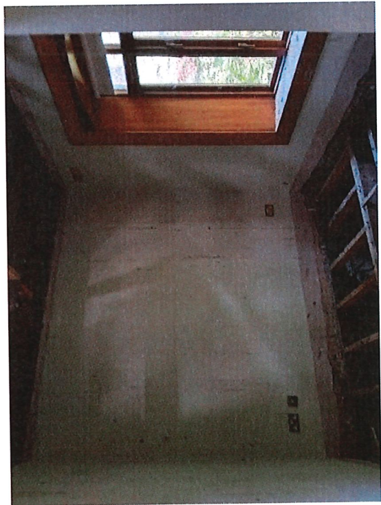
Fig. 4 - GF/02 - View northeast
