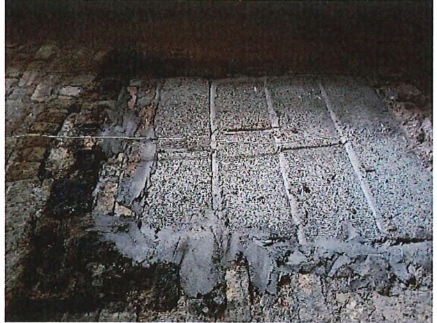
Fig. 11 – GF/05 – Detail blocked-up fireplace
