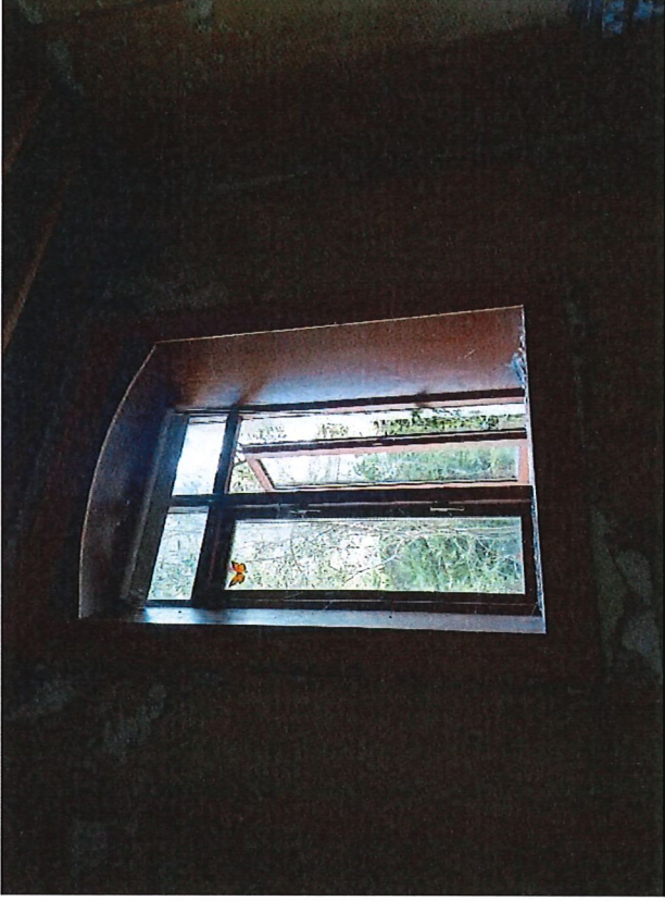
Fig. 10 – GF/05 - View east
