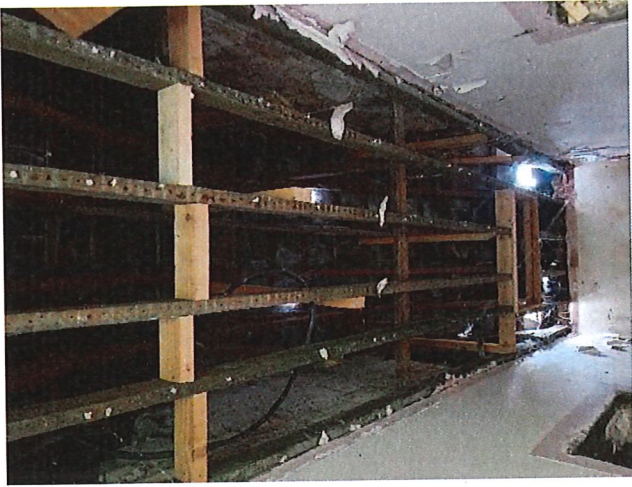
Fig. 3 - GF/01 - View roof internal
