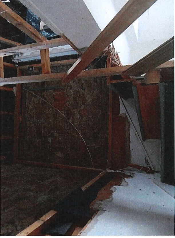
Fig. 4 – Coach House – F01/01– View east, stairs
